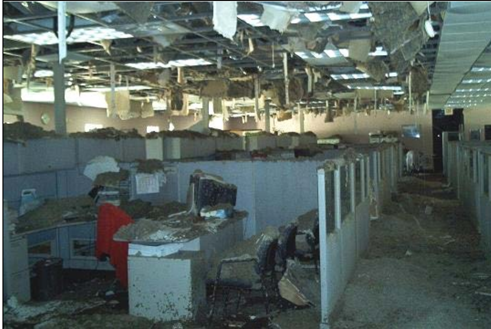
Figure 6: Inside the Kenner, Louisiana, District Office
